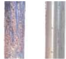
No Chemical BOILERMATE®
